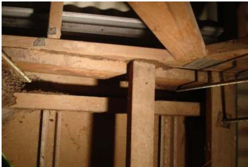
*Termite 'mud' packed in between framing timbers as well as a big mass of 'mud' on the left of the photo.*
