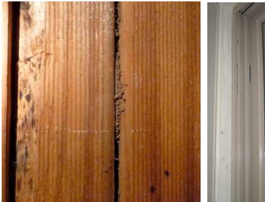
*Left: 'Mud' packed between two wall studs in an un-sheeted downstairs laundry. Right: Look carefully to see the 'mud' in the joints of the mouldings of this door frame and also see the uneven surface toward the top of the architrave where termites have come so close to the surface they've only left the thickness of the paint.*
