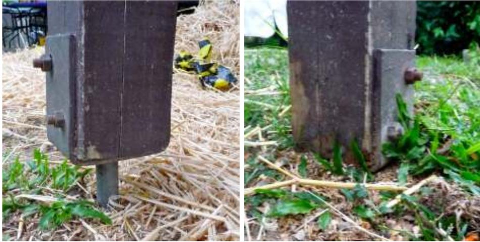
*Both these pergola posts are on galvanized stirrups. During your inspection you could see if a termite tunnel went up the stirrup on the right. The lawn surface has been built up to the post on the left and termites could go up the middle of the post and then across to the house.*
